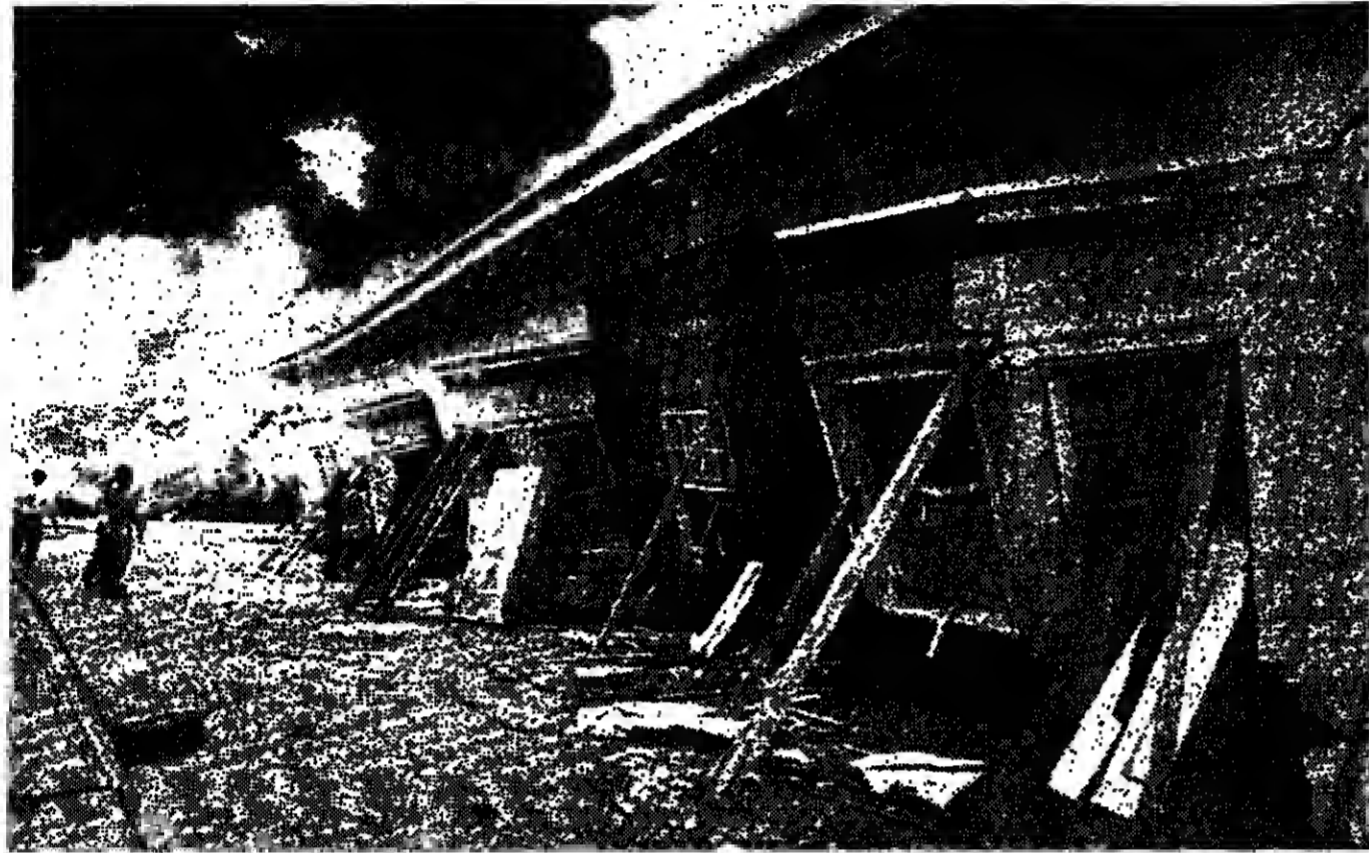
The remains of three-story buildings are propped up in the street in San Francisco's Marina District after sliding off their foundations and collapsing. Gas-fueled fires are raging in the distance of the blocked streets.
